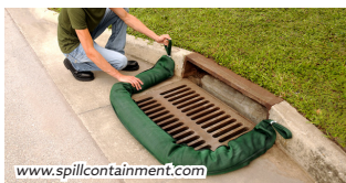
Inlet protection on a storm drain.
