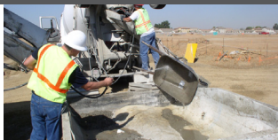
Roll-off system for concrete washout.
